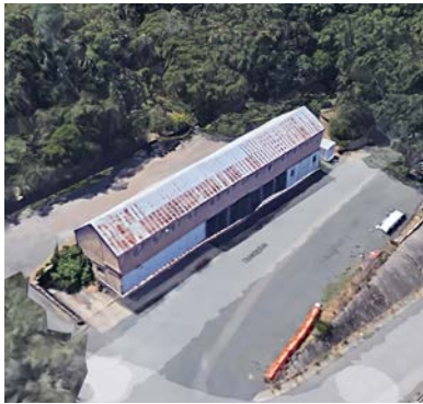
12 Boiler/Chiller Plant/Power House 7,515 SF Specific Plan Land Use: Flex Zone
