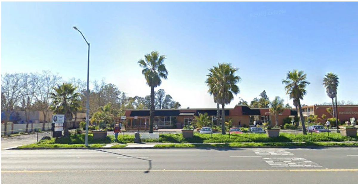
Figure 4.1-31 SAN-4 from Santa Rosa Avenue, Looking West
