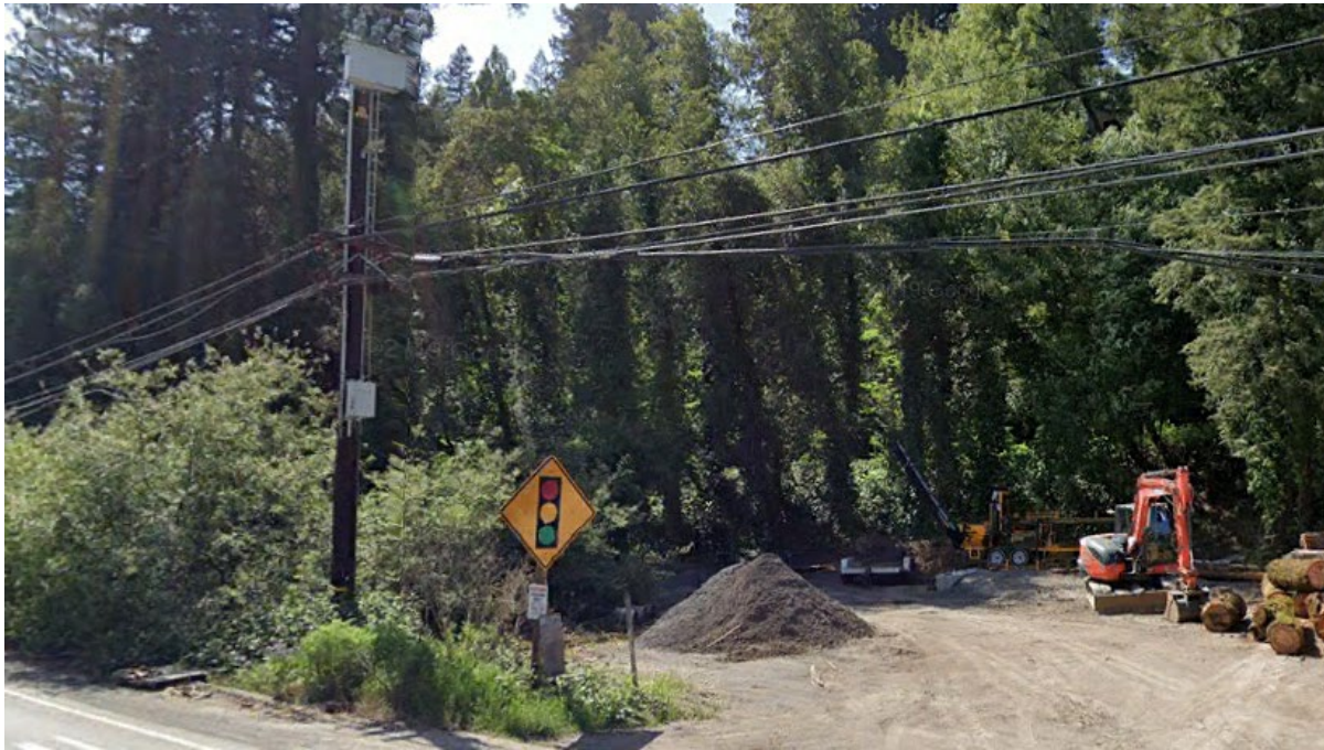
Figure 4.1-4 Site GUE-1 from River Road, Looking West Past Construction Stockpile
