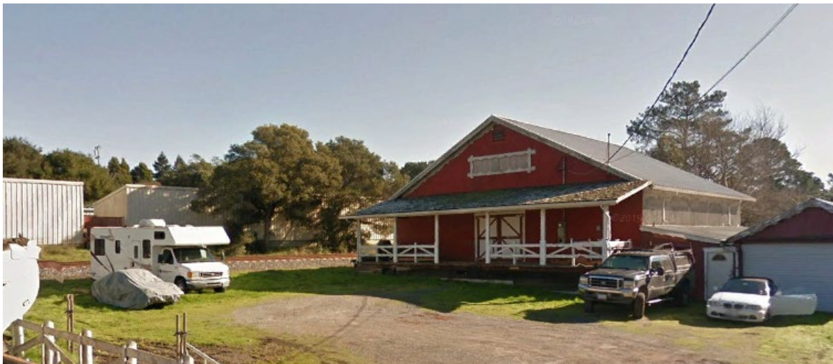
Figure 4.1-42 PEN-9 Looking Southeast
