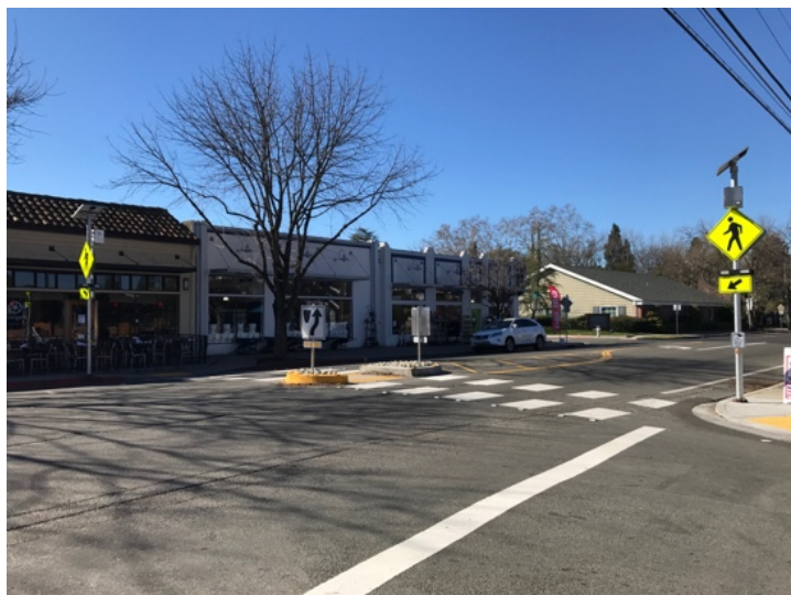
Pedestrian warning beacons with median refuge
