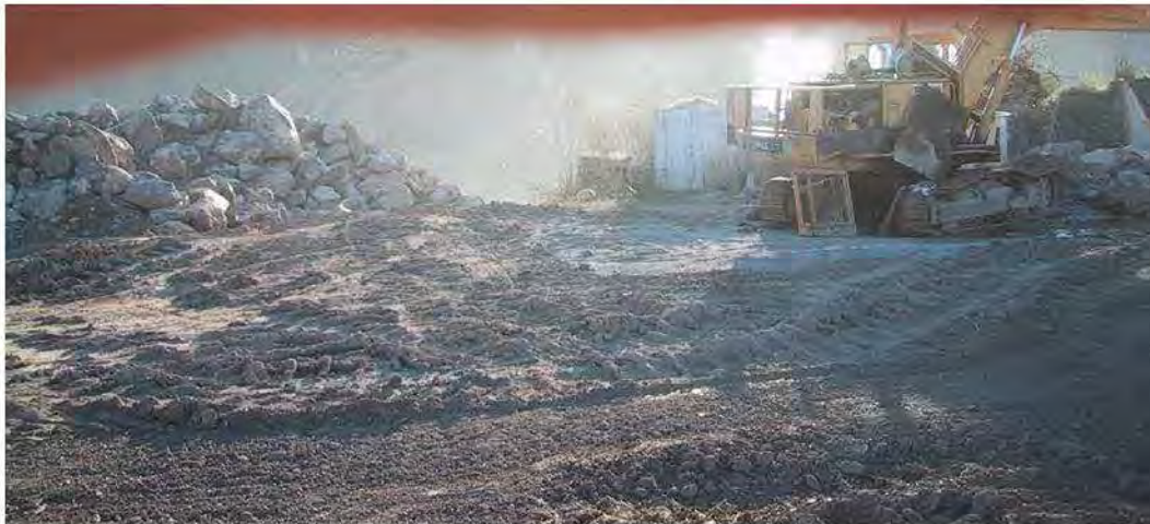
Figure B5: Short-Term Noise Measurements on Quarry Floor – Location ST5 & ST 6
