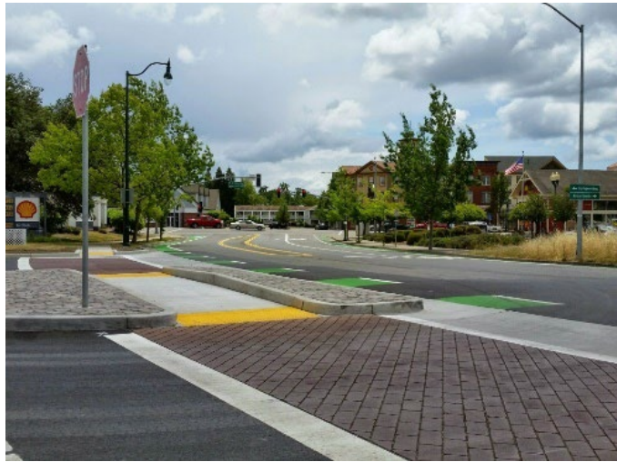
Intersection with pedestrian refuge, enhanced crosswalk markings and texture, and green bike lanes.
