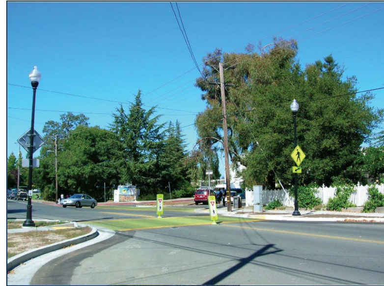
Clearly defined crosswalks and features such as bulb-outs increase pedestrian visibility to vehicles.
