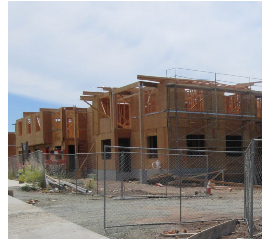
Fetters Apartments construction photo.
