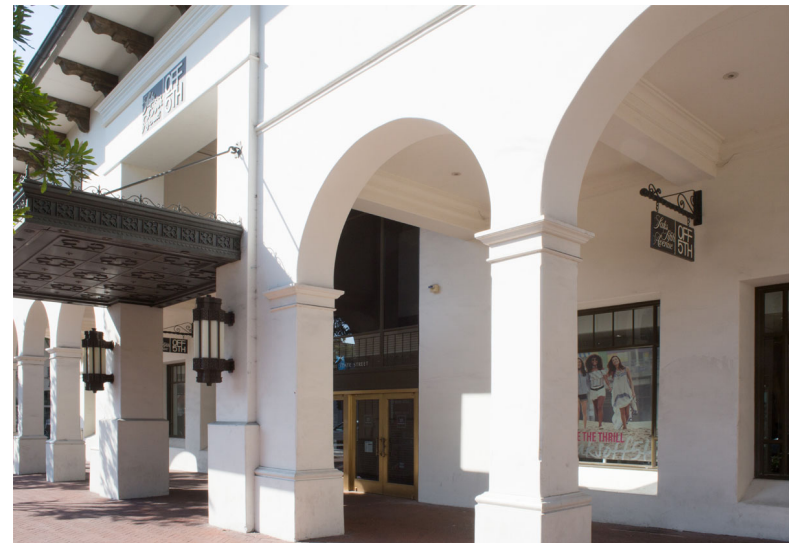
This arcade provides protection from the elements, while the recessed area and vertical elements create a pedestrian-friendly scale.
