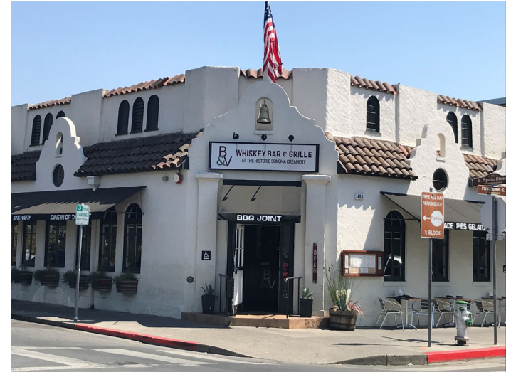
This building is oriented toward the street corner with the primary entrance, located on the diagonal, easily visible and accessible. The larger mission façade and mission bell distinguish the entry from other elements of the building.
