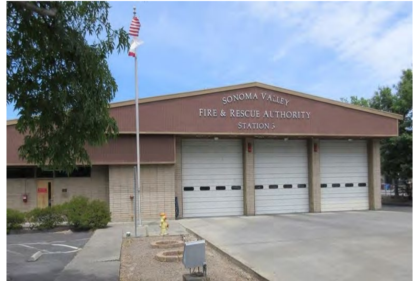
Sonoma Valley Fire and Rescue Authority Station 3, located northwest of the intersection of Agua Caliente Road and Highway 12.
