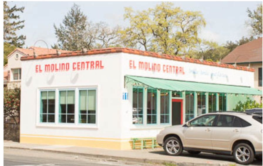
Ground-level windows facing sidewalk and parking area create an inviting street-front for pedestrians and a welcoming façade and the pedestrian-scale awning enhances the building entrance.
