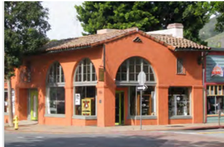
In this example, the color scheme uses a single base color for building walls and a single accent color for windows and doors.
