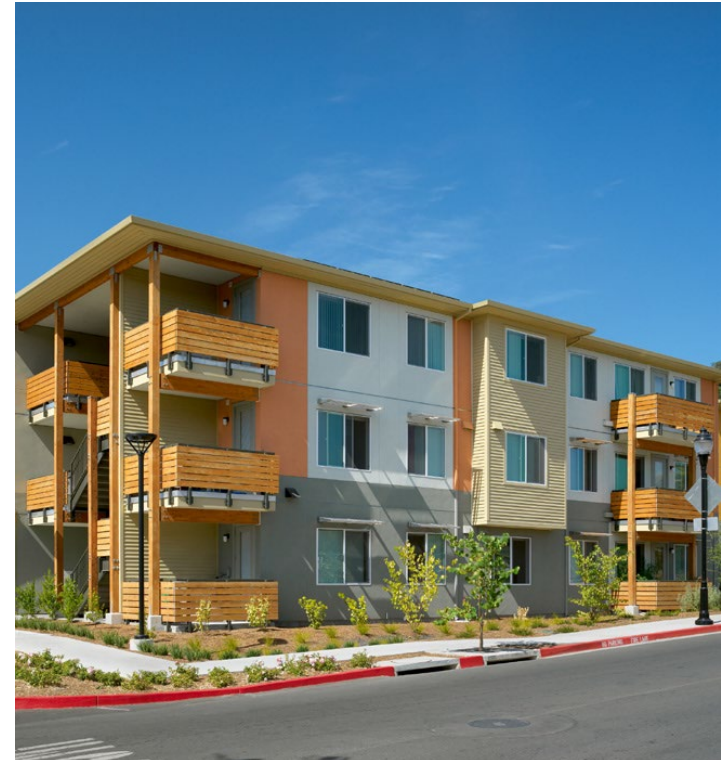
Fetters Apartments provides housing affordable to the local workforce and seniors. The MidPen development includes a community garden, shared playground with Sonoma Charter School, and space for community supportive services. (Photo source: MidPen Housing)
