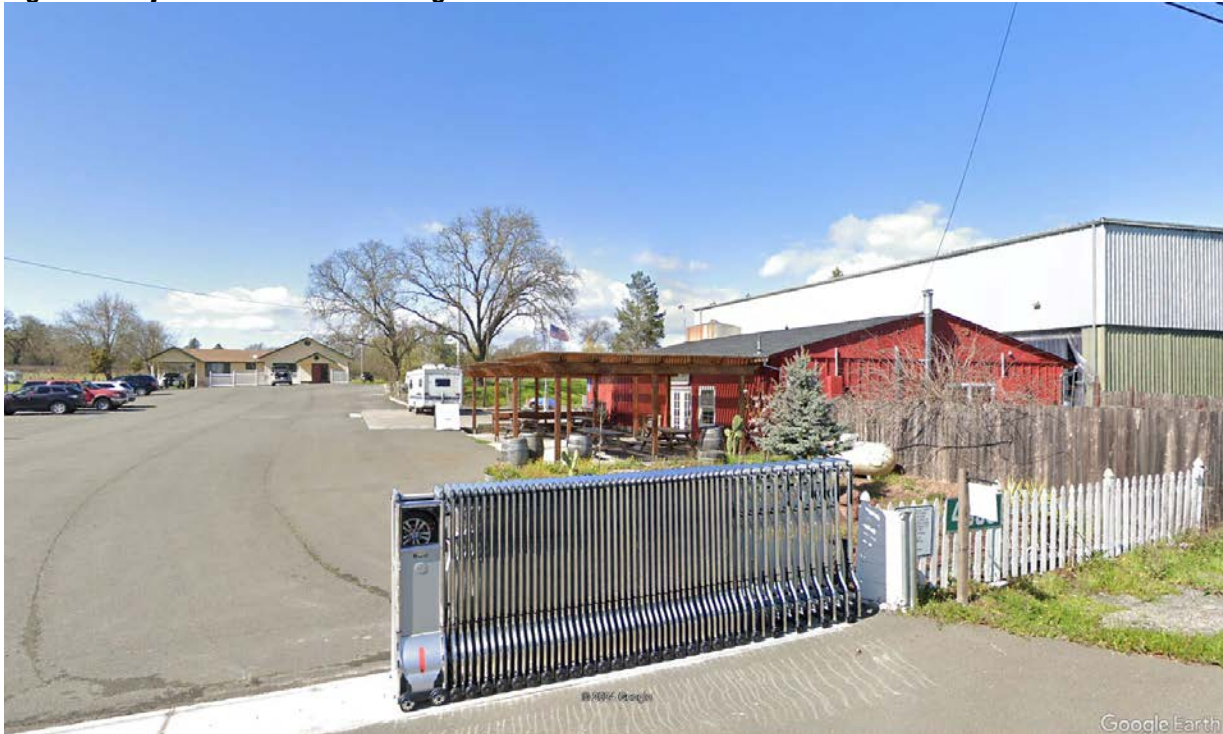
Figure 4. Project Entrance and Parking Area
