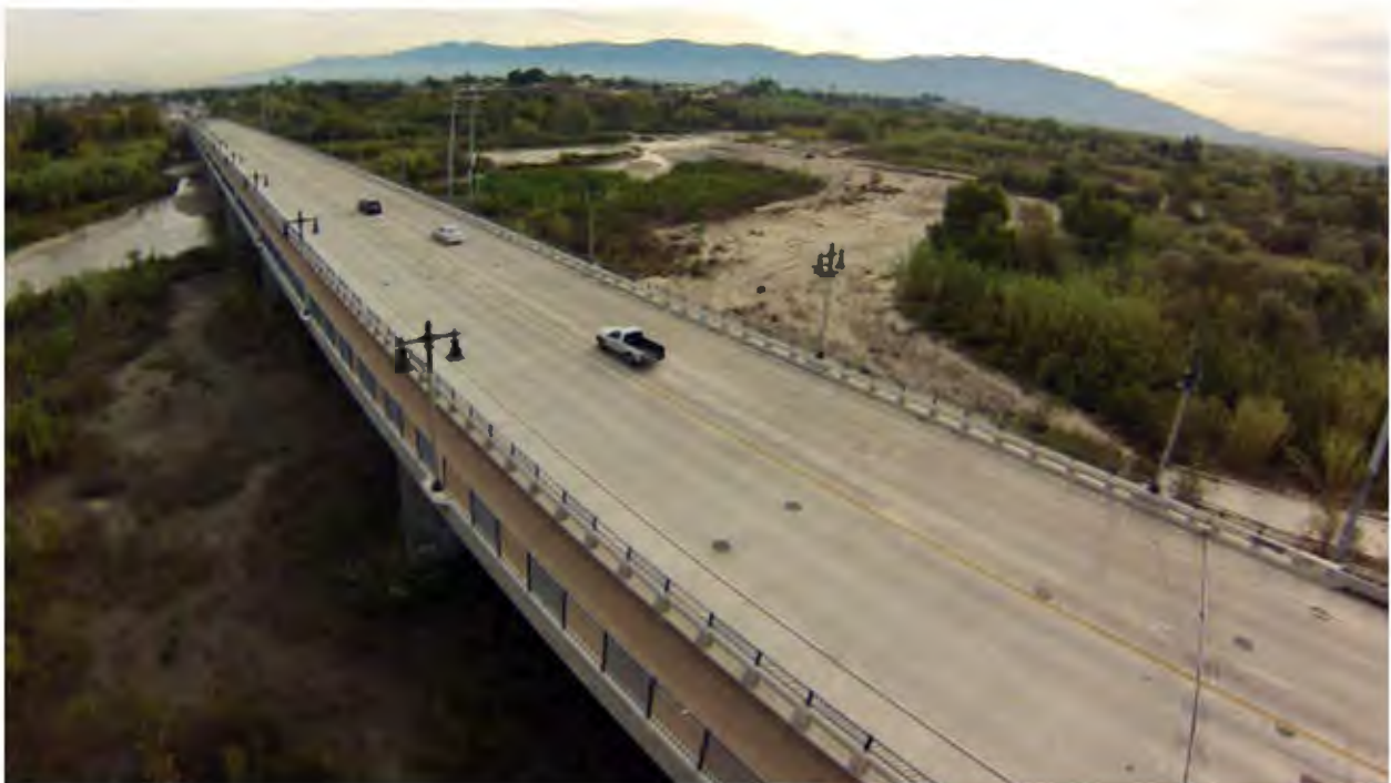
Figure 9 Image of Completed River Road Bridge (After Construction)
