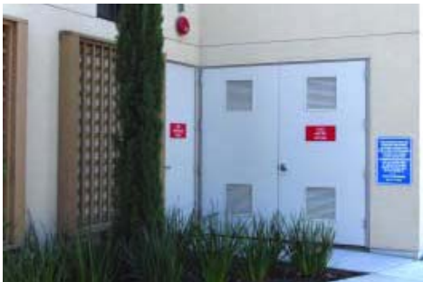
It is recommended that buildings be designed to include locations for mechanical equipment within the building itself.
