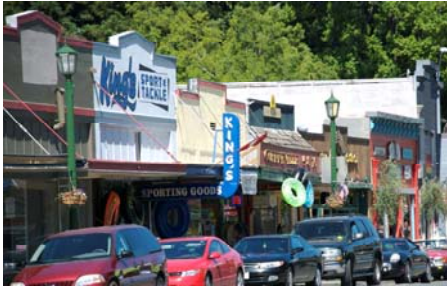
Many buildings in downtown Guerneville feature a false front capped with a shaped parapet or cornice.
