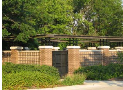
Commercial dumpsters and mechanical equipment have been located adjacent to the parking area and screened by an architectural wall and landscaping.
