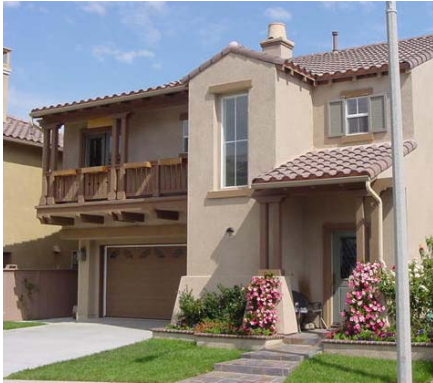
A garage door set back from the face of the house reduces its visual dominance.
