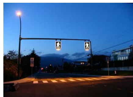
Illuminated crosswalks improve pedestrian safety.
