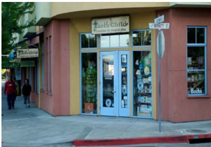
Color, transom windows, and sidelights are used to enhance this corner entrance.
