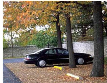
Traditional pavement is used for the travel lanes in this parking lot while car stalls are constructed of porous pavers to allow for better root growth.
