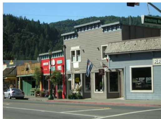
Commercial buildings located along Guerneville's Main Street.
