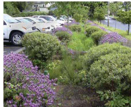
This vegetated swale captures storm water runoff from the adjoining parking area.
