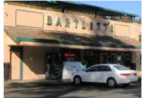
The attached wall sign of Bartlett’s grocery store in Monte Rio consists of individual, three-dimensional letters.
