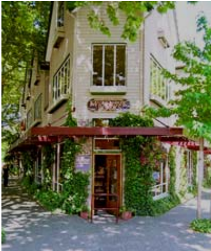
This building capitalizes on its unique corner location by providing a corner entrance which is accentuated with a transom window, canopy, and planters.
