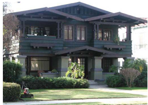
This quadplex has the appearance of a single family residence and is designed to complement the neighboring residential uses.
