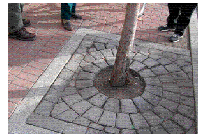
Pavers may be used in tree wells to allow infiltration of rain water and to extend the walking surface of the sidewalk.
