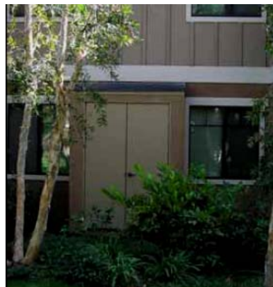
Utility meters are enclosed within a cabinet that blends with the building's architecture.
