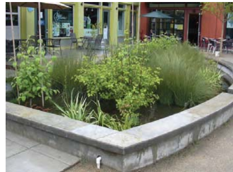
Infiltration planters have open bottoms to allow storm water to slowly infiltrate into the ground.
