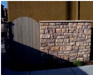
A masonry wall and wooden gate provide an attractive means of screening utility equipment.
