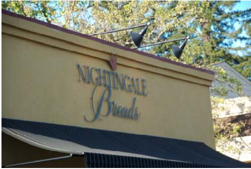
Gooseneck lamps are the preferred method of illuminating attached wall signs.
