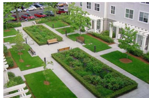
Infiltration basins are provided in the courtyard of this multifamily development.
