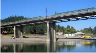
Monte Rio Bridge c. 1934.
