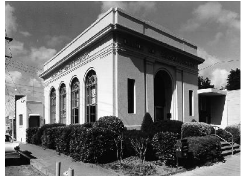
The Bank of Guerneville is the sole example of Beaux-Arts architecture in the area. Constructed around 1920, the building features a flat roof with an accented wraparound cornice. The arched entrance is flanked by pilasters and a fanlight is located above the wood doors. Four full-height arched windows adorn the side of the structure.
