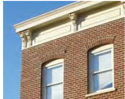
A projecting cornice accentuates the parapet of this building.
