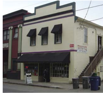
Residential units are located above the retail space of this mixed-use building.
