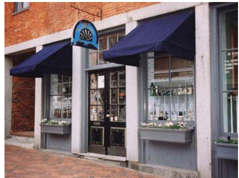
Awnings are fabric elements which project from the building facade above the windows or doors.
