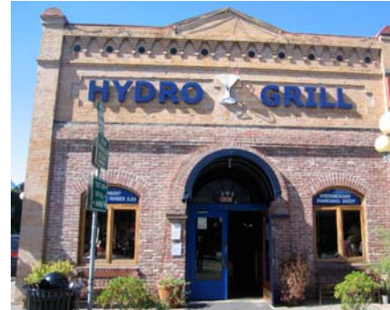
Attached wall sign placed within a recessed molded band that has been incorporated into the building's design.
