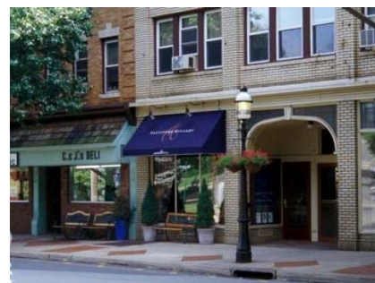
Recessed entries are a common feature of a traditional Main Street storefront.
