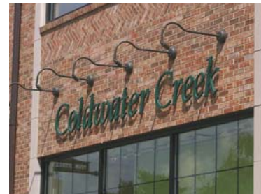
Gooseneck lights are used to illuminate this attached wall sign.
