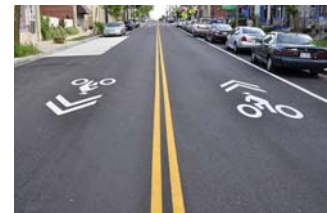
Shared-use arrow (Sharrow) pavement marking.
