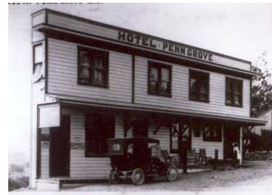
Hotel Penngrove constructed in 1906.
