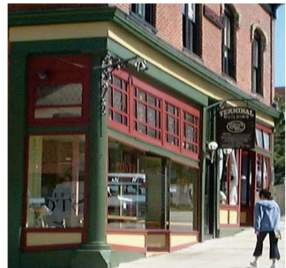
Transparent windows provide a visual connection between pedestrians and the building's interior encouraging potential customers to enter the shop.
