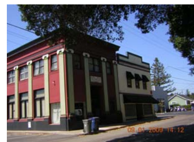
The bank building, constructed in 1922, stands next to the Evert building (pictured above).
