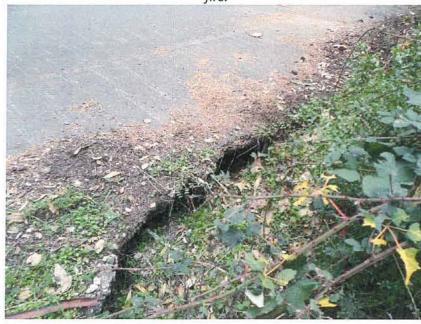
**Photo 24**: Undermined area beneath the pavement at Moon Watch Lane. To be backfilled & compacted with base rock and ripraps up till finished grade
