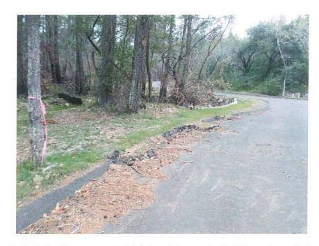
Photo 1: Significant amount of debris and damage to the AC Berm towards the Northern corner of Lot 12. Needs to cleared and repaired.
