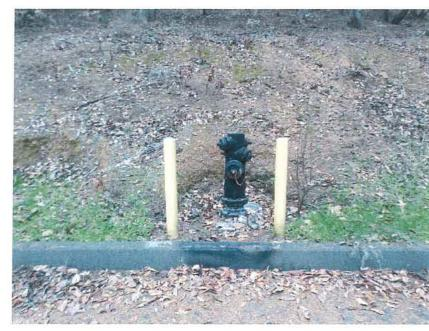
**Photo 21**: Fire hydrant at the turnaround near Lot 11 damaged during fire.
