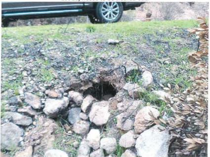
Photo 11: Inlet to be monitored for silt collection to avoid blockage.
