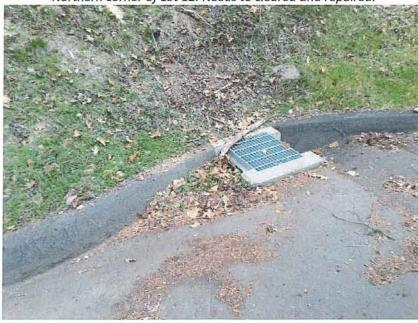
Photo 5: Collection of leaves and debris blocking the drainage path along the driveway near Lot 2. Needs to be cleared out.
