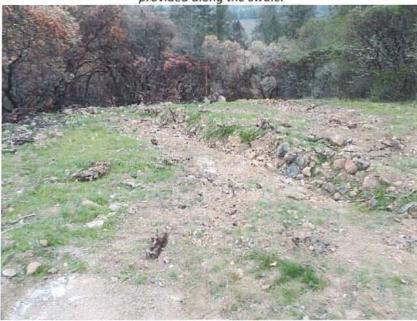
**Photo 29**: Water bars near the slopes around the proposed inn location appear to be adequate thus no improvements required. Monitor monthly or after significant rain event.
