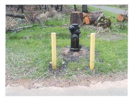
**Photo 16**: Fire hydrant near the south junction of Lot 7 damaged by fire. Needs to be power washed or repainted.
