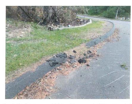
Photo 2: Significant amount of debris and damage to the AC Berm towards the Photo 3: Damage observed along the AC Berm towards the Southwest of Northern corner of Lot 12. Needs to cleared and repaired.
