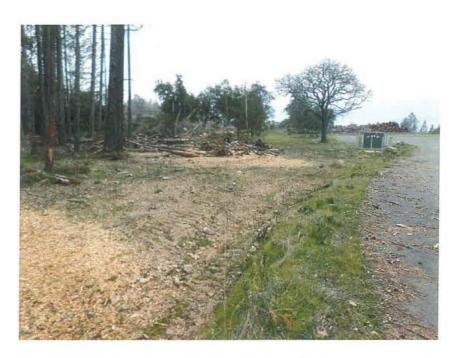
**Photo 26**: Fallen branches and debris to be cleared and straw wattles to be provided along the swale.
