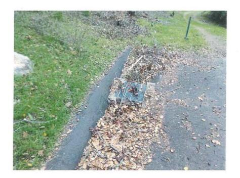
**Photo 7**: Collected debris near the Drain Inlet near the turnaround at Ten Oaks Way needs to be cleared out.
