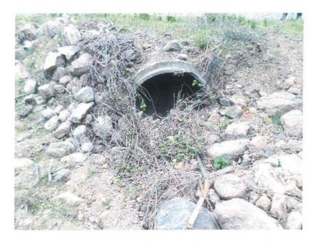
**Photo 25**: Culvert near the end of Campagna Lane obstructed with debris, need to be cleared out.
