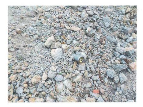
Photo 13: Property corner near the dirt road at lot 7 damaged.
