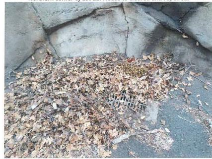
Photo 4: Collection of debris above the drain inlets near the southern side of Lot 4. Needs to be cleared out to avoid blockage.
