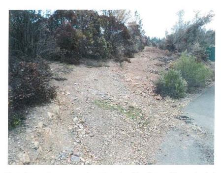
**Photo 14**: Provide straw wattles at the edge of the dirt road & near the drain inlet to avoid erosion.
