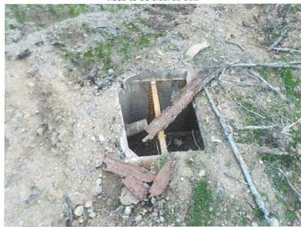
Photo 28: Utility box damaged and needs repairs and replacements.
