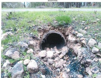
**Photo 18**: 27" culvert pipe near the junction observed to be damaged during the fire. Top needs to be repaired and remove melted plastics.
