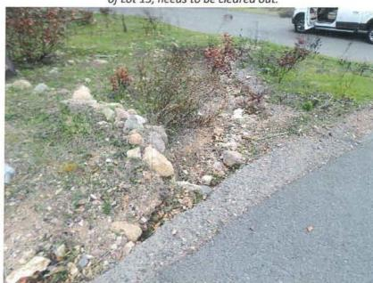
**Photo 12**: Erosion observed near the driveway leading to the water tank.
