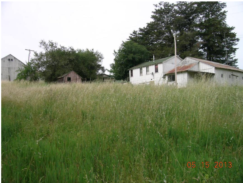
Figure 5. Winery location will be within the grasslands in the foreground. The buildings on the right will be renovated as well as the barn in the background.
