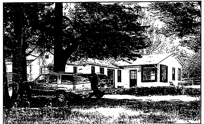
Figure 2. Building 2, west elevation.
