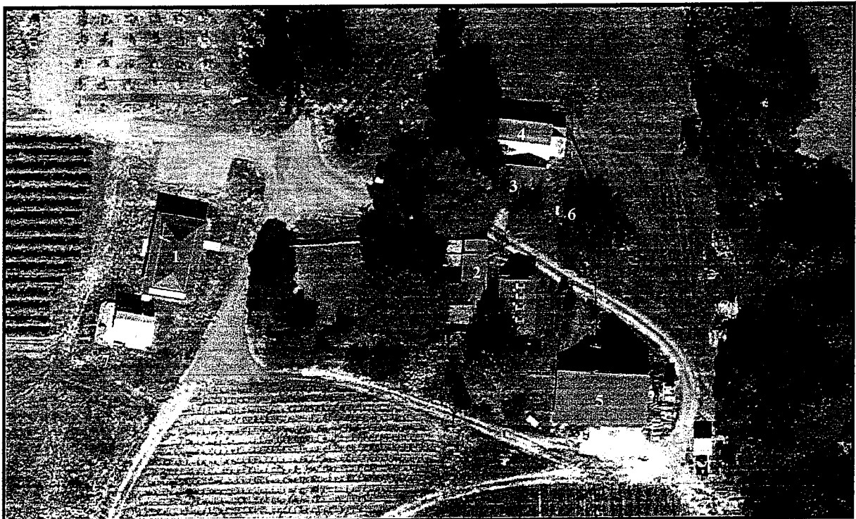
Figure 5. Aerial view of the Belden Barns complex.
