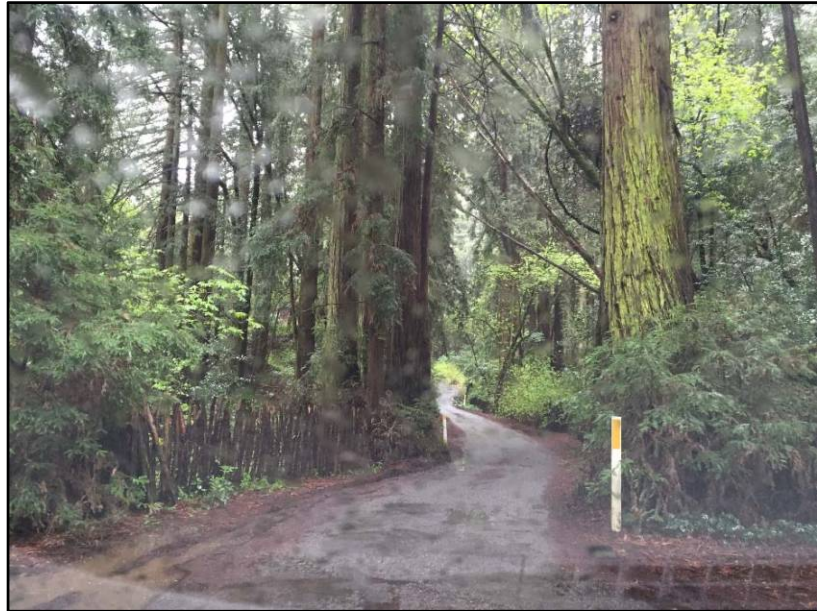
Photo 3 – Narrow pavement and vegetation on both sides of the Sonoma Mountain Road
