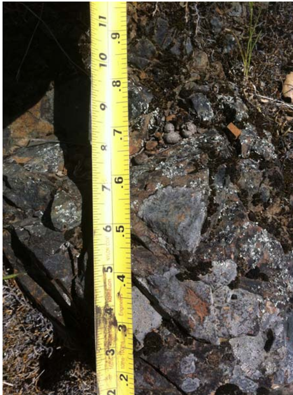
Photograph 5 Close up view of typical weathered rock outcrop in the upper portions of the slope. Fracture spacing and orientation appears to result in the majority of rock fragments being 8 inches or less in maximum dimension.
