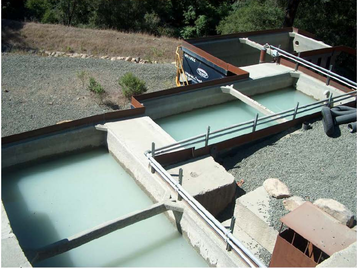
Appendix G5. Drainage E1 sediment detention features, Mark West Quarry, Sonoma County.
