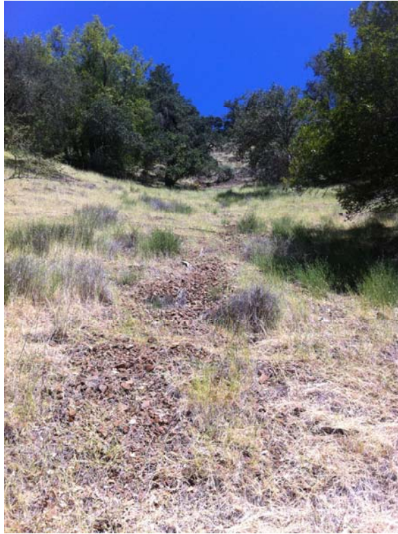
Photograph 3 Lower portion of slope showing accumulated gravel-size rock fragments and very thin surface vegetation.
