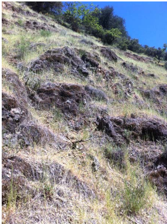
Photograph 4 Typical weathered rock outcrop in upper portions of slope.
