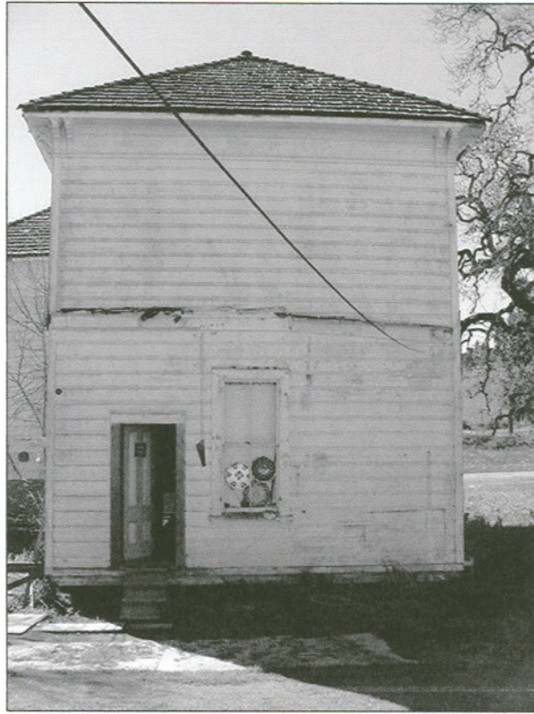
Figure 5. East Side of House
