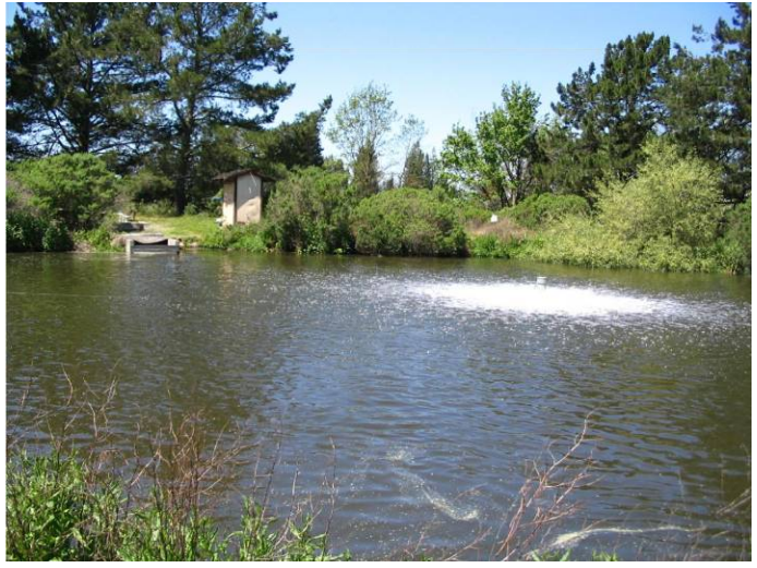
WWTP AERATION POND WITH STORAGE SHED IN BACKGROUND
