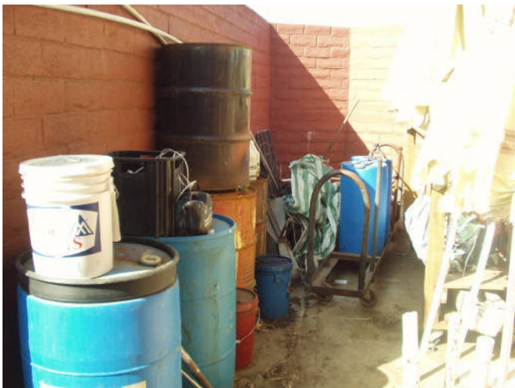
View of chemical storage area outside of the LBC Physical Plant building.
