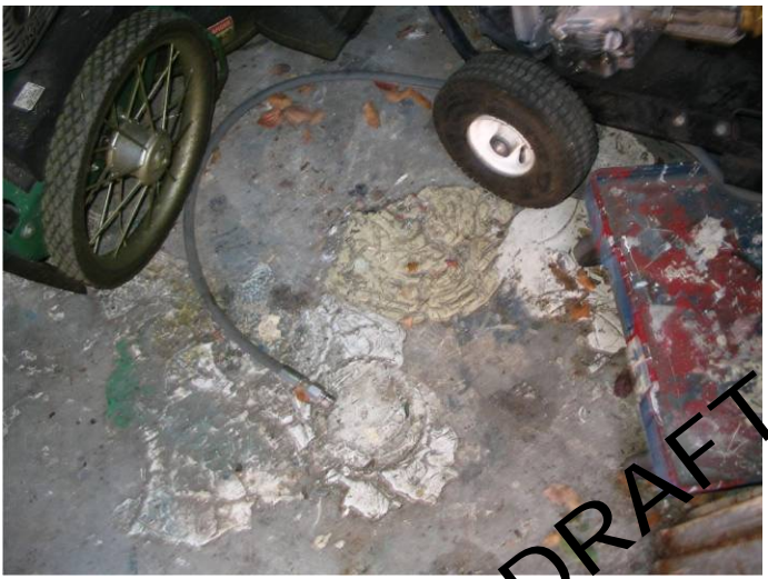
PAINT SPILLAGE- PHYSICAL PLANT BUILDING UTILITY CLOSET
