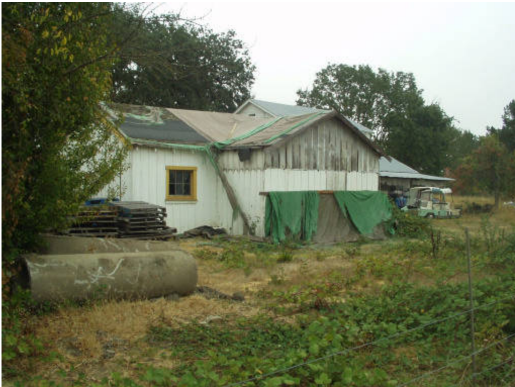
View to the east of the garage building within the homestead property.
