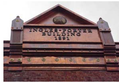
A building identification sign acknowledges the historic
