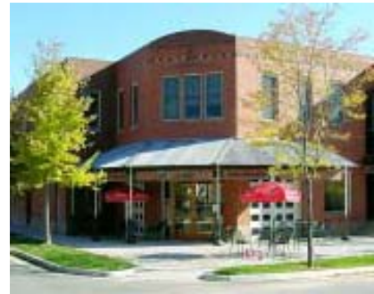
This building has been designed to capitalize on its prominent street corner location by providing a corner entrance and accentuating the corner portion of the building with an awning.
