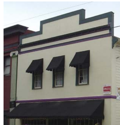
The false front of the Ewart building features a parapet.
