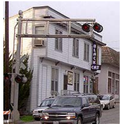
Originally constructed in 1906 as a hotel, this two-story flatiron building features horizontal wood siding.
