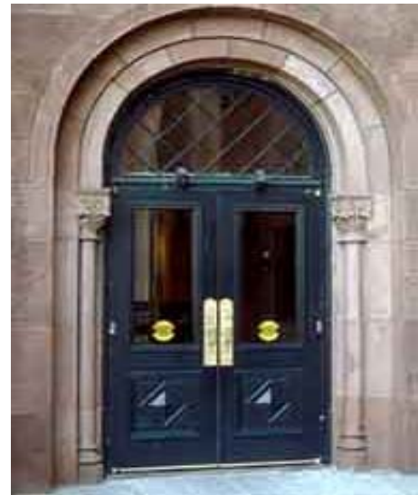
An automatic door provides a practical means of meeting accessibility requirements.
