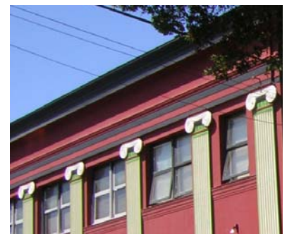
The 1922 bank building features a parapet with a projecting cornice.
