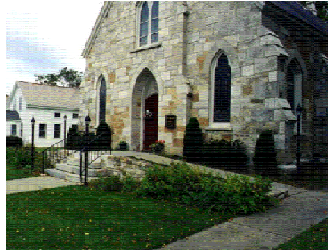
An accessibility ramp should be compatible with the historic building in terms of scale and materials. The historically significant front stairs of this structure were pulled forward to allow space for a side access ramp. The low wall in front of the ramp is constructed of masonry which matches the building.
